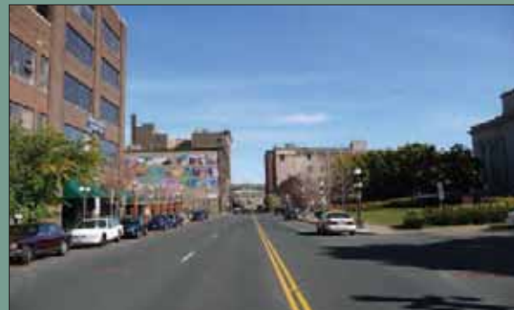
05: The alignment will continue along the south side of 4th Street in front of Union Depot. The Union Depot Station will abut the existing front lawn of the station.
